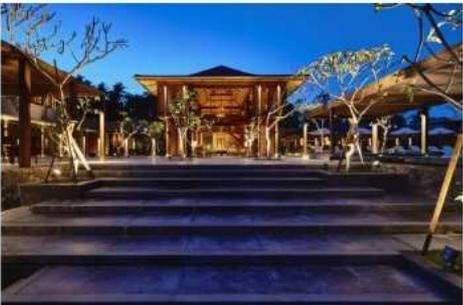
The main structures, which house the living areas are built as double height timber frame structures, clad in louvered shutters which allow for natural ventilation – avoiding air conditioning in these areas – and creating a rich play on light at night.
