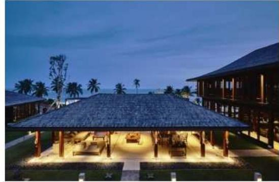
The roofs are parallel to the slope, they are simple angled rectangles in clay tiles. They extend out to cover the walkways and are held up, on the open side, by a long series of V shaped timber columns. These create the 'outside' skin of the building and establish a strong rhythm along the facades. At the back of the studios another single building houses the kitchen, outdoor dining and washrooms.
